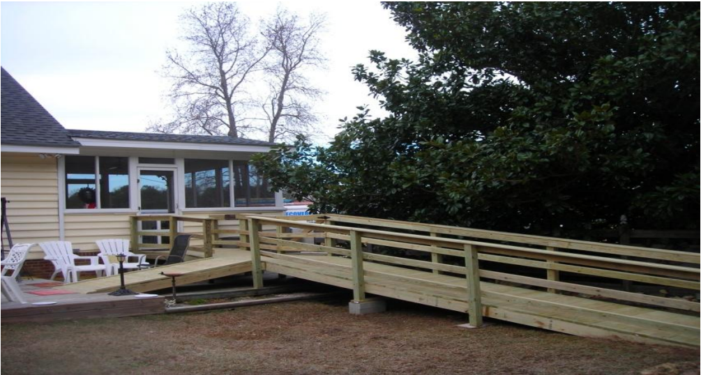
This is a partial view of a Straight Ramp with a little kicker ramp to the side. So this dear lady could get down to her deck and still be able to enjoy a spring afternoon on her back deck.
